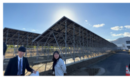
PPA bifacial solar panels in school lunch facilities
